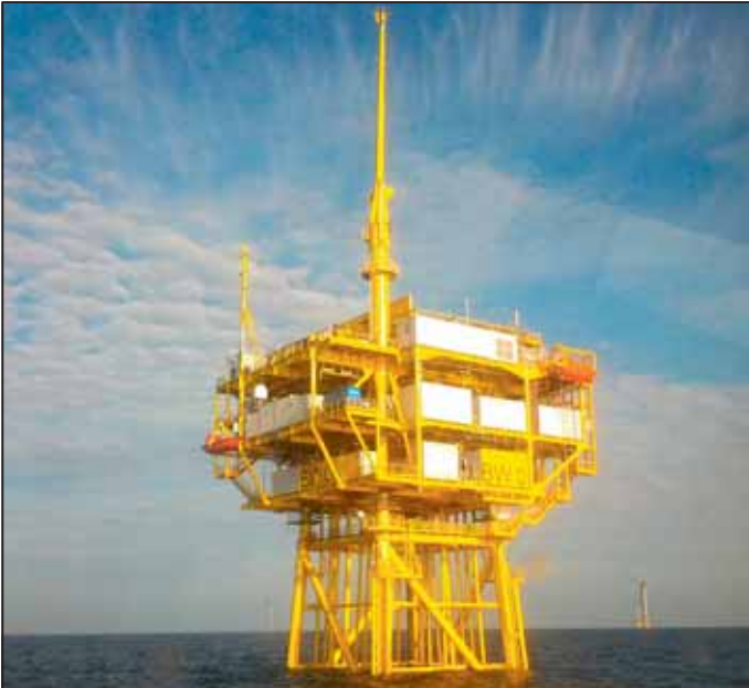
Umspannplattform im Windpark Borkum West 2 Transformer platform in the wind park Borkum West 2
